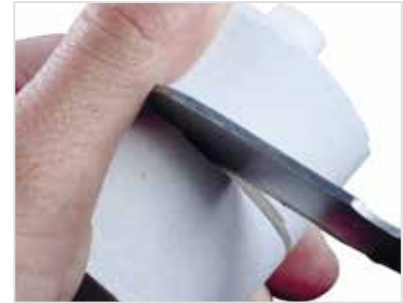
c) With a plaster knife, break at the incision.
